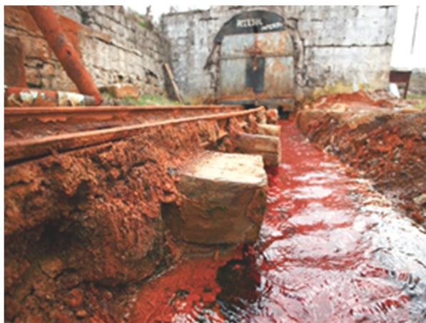
Fig. 1. Water drainage at “Gura Minei” abandoned mining perimeter (23.05.2014, A. Lancranjan)
