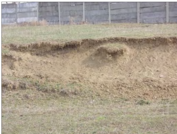
Fig. 1. Landslide in the proximity of the compressor station
