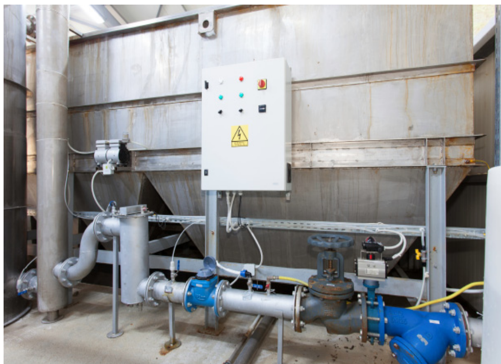
Fig. 5. The electrochemical pre-treatment stage within the water potabilisation station of Romuli township - Bistrița-Năsăud county
